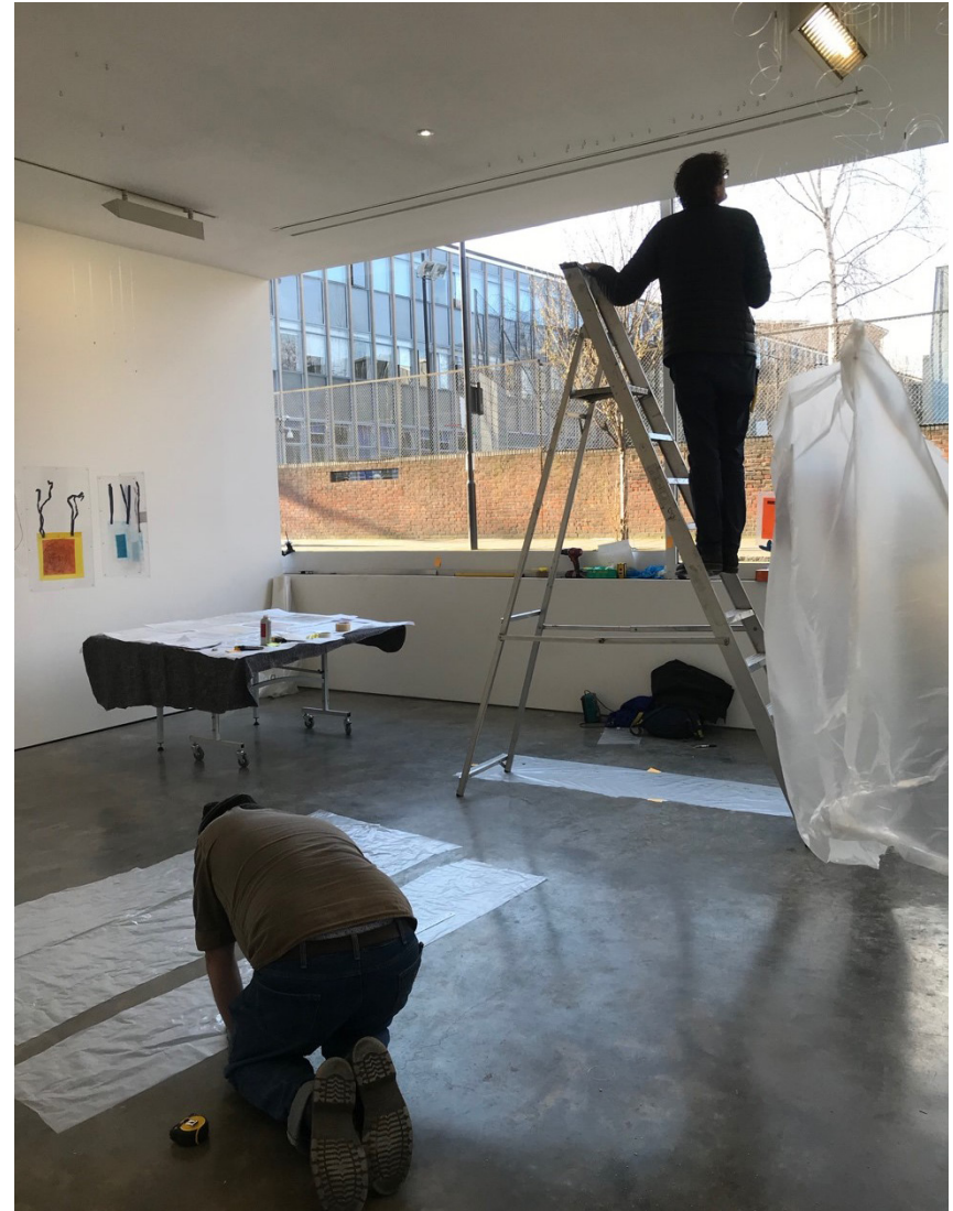
Fig.18 Installing Room 2 environmentpoem
